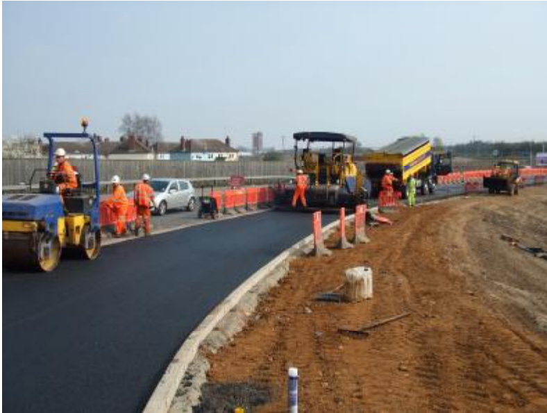
Surfacing at A47 approach
